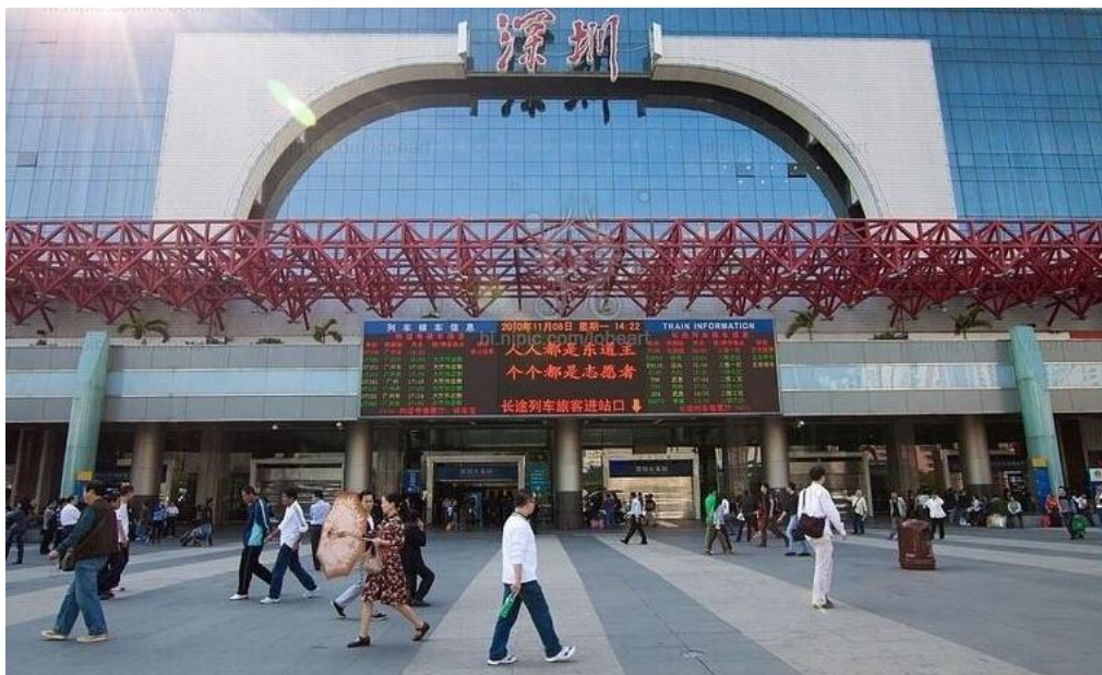
Shenzhen Luohu Railway Station
